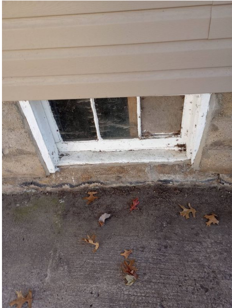
You can see significant leaning on this window under the carport
