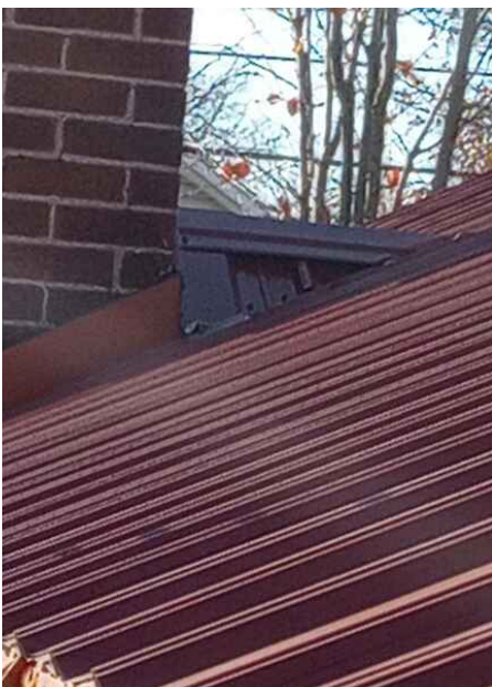
Flashing at Chimney
