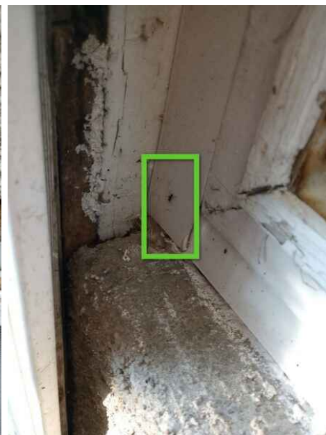
Window into crawl space. Ant
